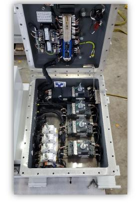
➤ The increased safety enclosure contains terminals and provides the interface between the flameproof panel and the installation wiring.
